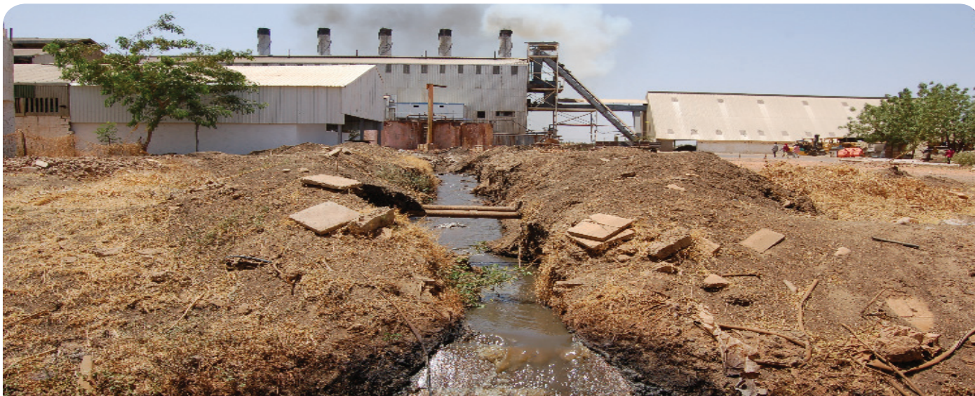
Untreated effluent flows from the Assalaya sugar factory into the White Nile, Sudan.
